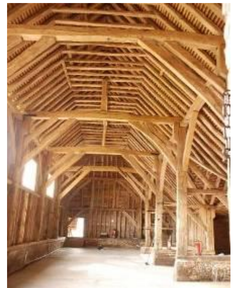
The repaired barn at Kingsbury Manor
