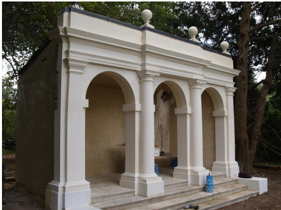
The finishing touches being applied to the repair of the temple
